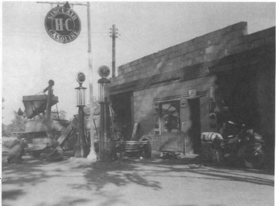
The Sinclair Garage and farm repair shop where I finally found my electrical problem. The owner is doing arc welding on a combine.
